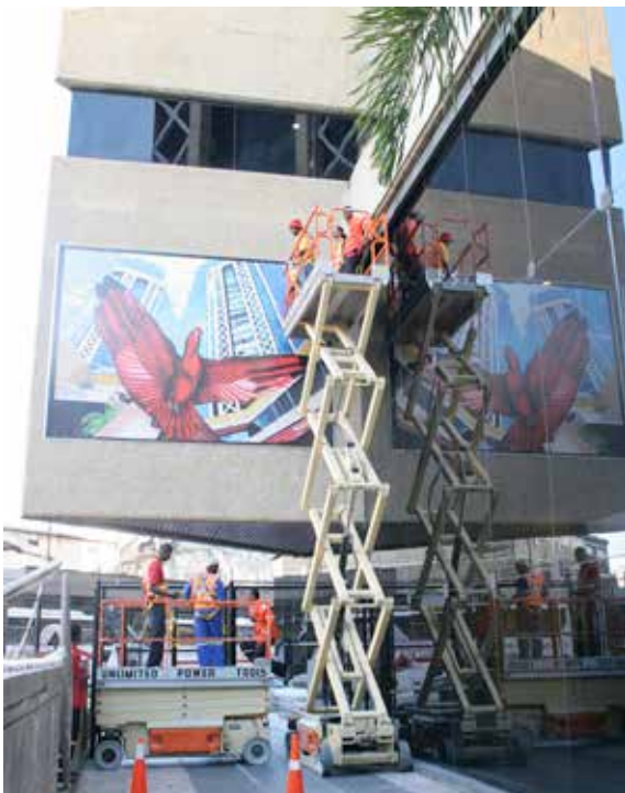
Mounting of the final piece of Art on the Wall project
